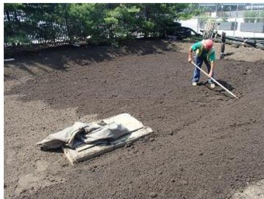
[An example of a bioinfiltration basin installation](#)
